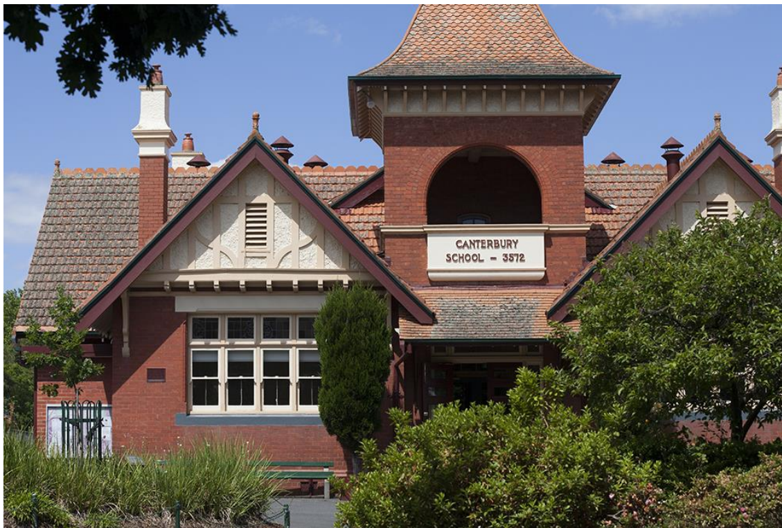
Canterbury State Primary School, Victoria
